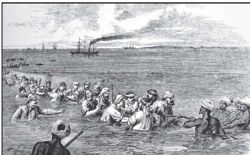
Figure 3: Laying of telegraph cable in the Persian Gulf (From https://atlantic-cable.com/ )
