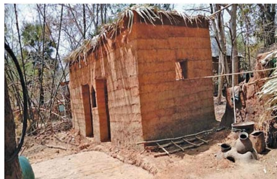
2. Mud house under construction
