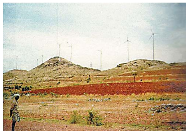
Fig. 16: Wind farm at Hiriya.
