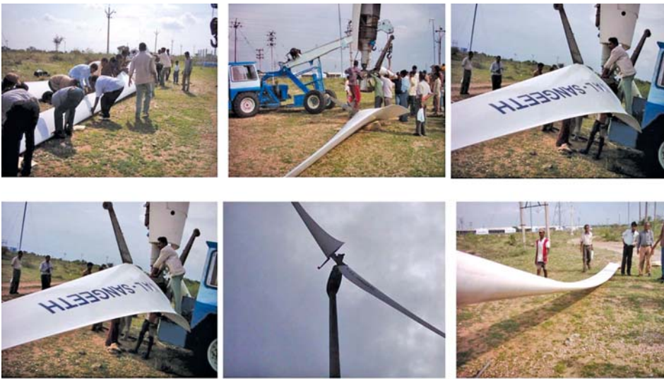
Fig. 17: Installation and commissioning of 300 kW wind turbine.
