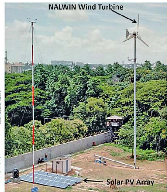
Fig. 21: 7.5 / 7.5 kW WiSH Technology Demonstrator at Kodihalli Campus, Bengaluru.
