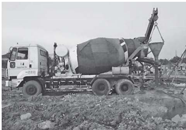
Fig. 1. Concreting in pile after erecting the steel cages, tremie shakings of concrete flow compact inside of pile bored holes.
