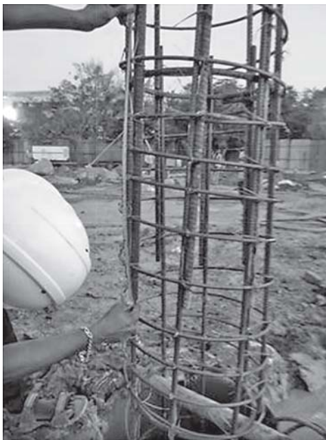
Fig. 4. Lapping connection check in erection process in boreholes.
