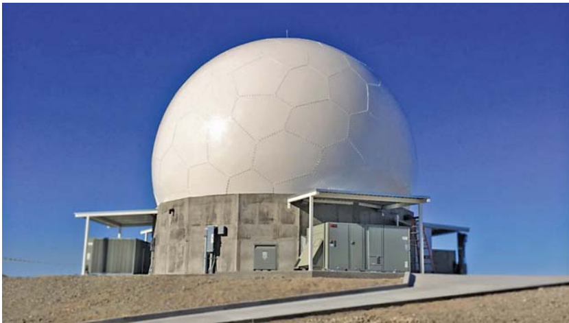
Fig. 1: Ground based radome (Courtesy: https://www.tcn.al/tcn/wp-content/uploads/2018/10/radome-1024x683.jpg )
